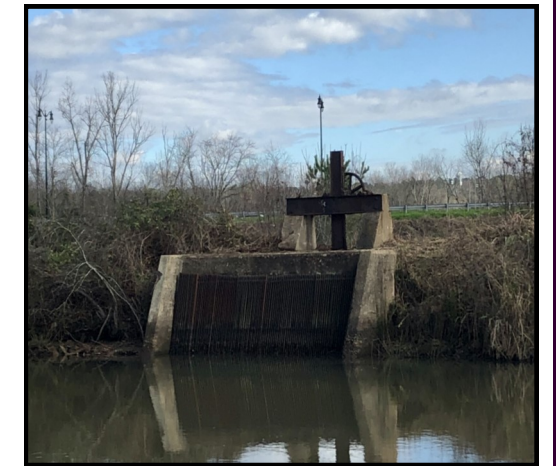
What is left of the Russell and Simmons mill. This is located just north of Sibley Mill, across the canal
